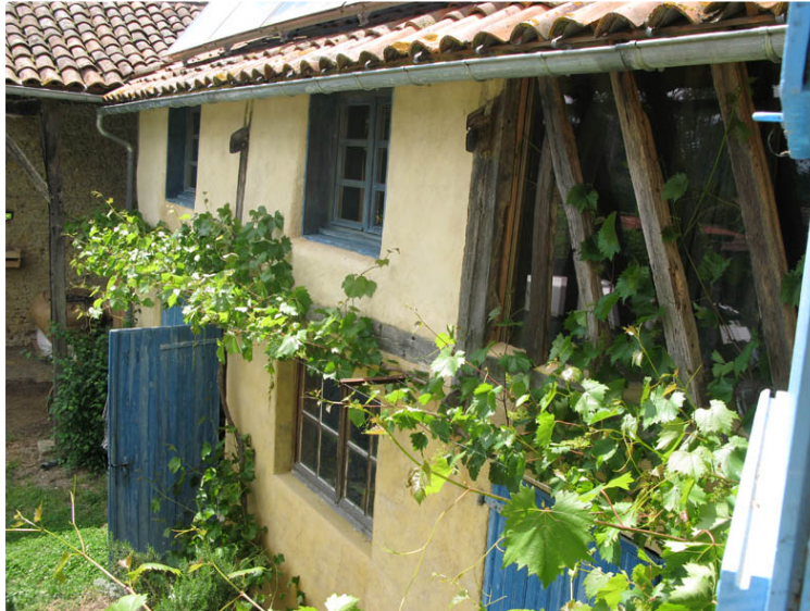
RISCLE ECO CONSTRUCTION
